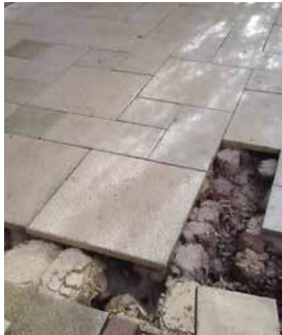
Spot bedding giving poor support
